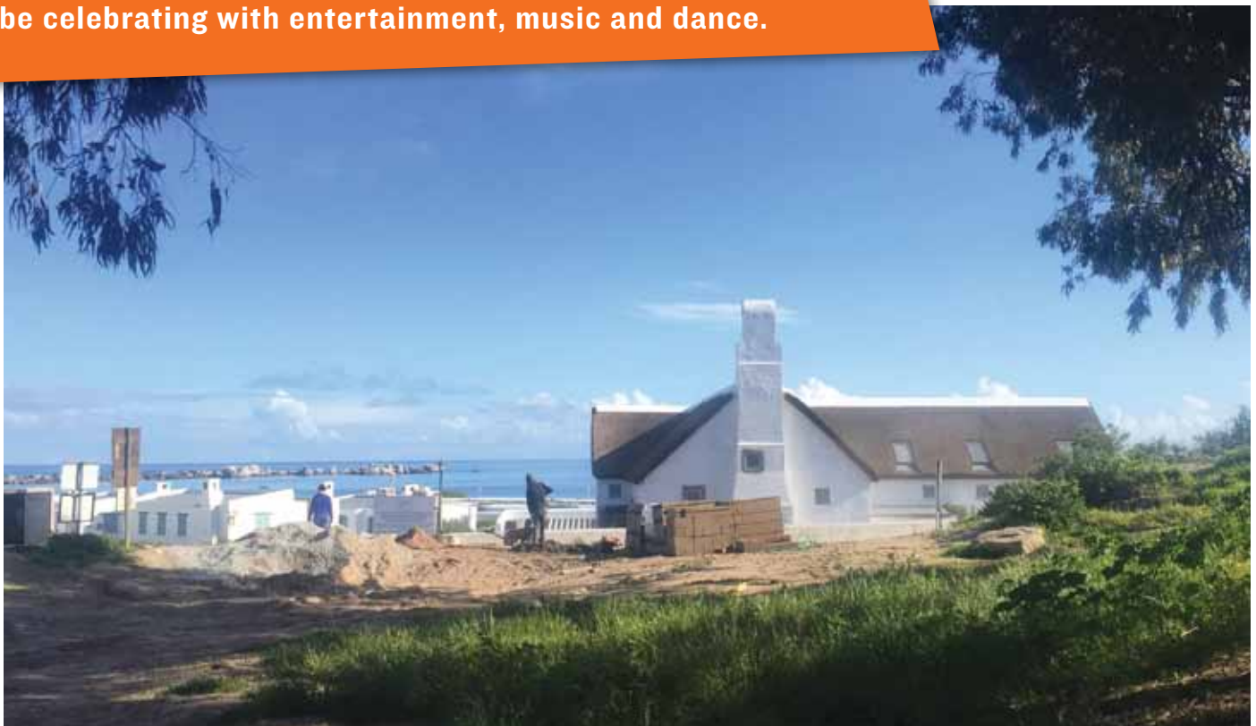
The Volunteer House nearing completion.
